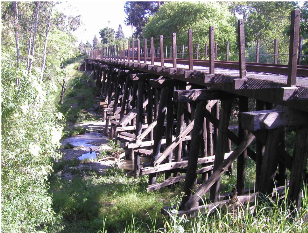
Fig. 4: View of the Trestle from the planned Los Gatos Creek Trail
