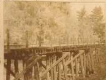
The train trestle on a trail in San Jose's Willow Glen neighborhood was saved from early demolition by a judge ruling that the City Council's 2008 plan to demolish it was unconstitutional. An environmental impact report for the bridge is due.
