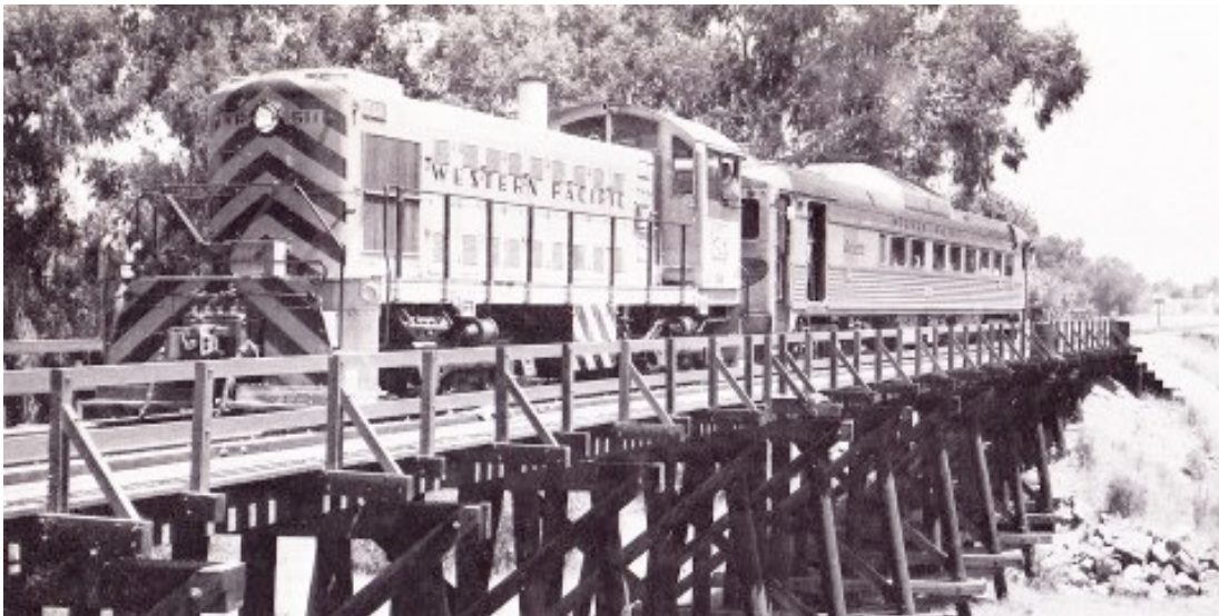
The Willow Glen Trestle in 1955
