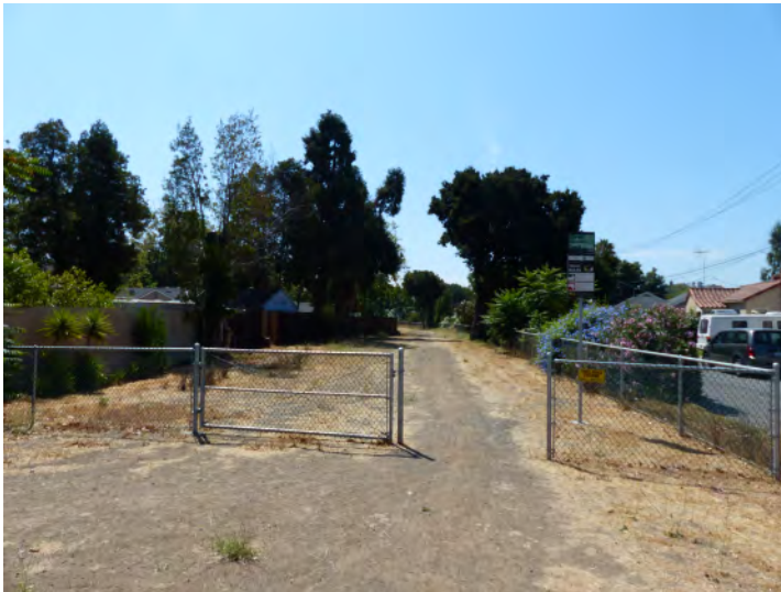
Photo 7. View of trail entrance Coe Avenue facing southeast.
