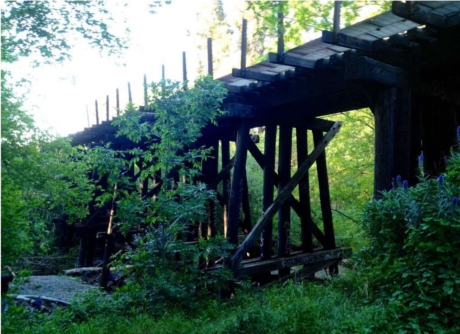
View of the Willow Glen Trestle from 2014, viewed from the southwestern side, the site of a proposed viewing area.
